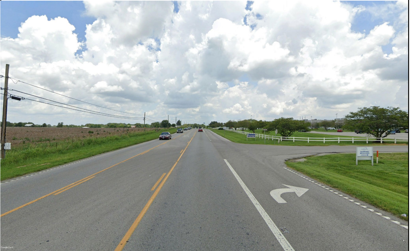
Previously widened section of US 31 W near Franklin Precision Industries
