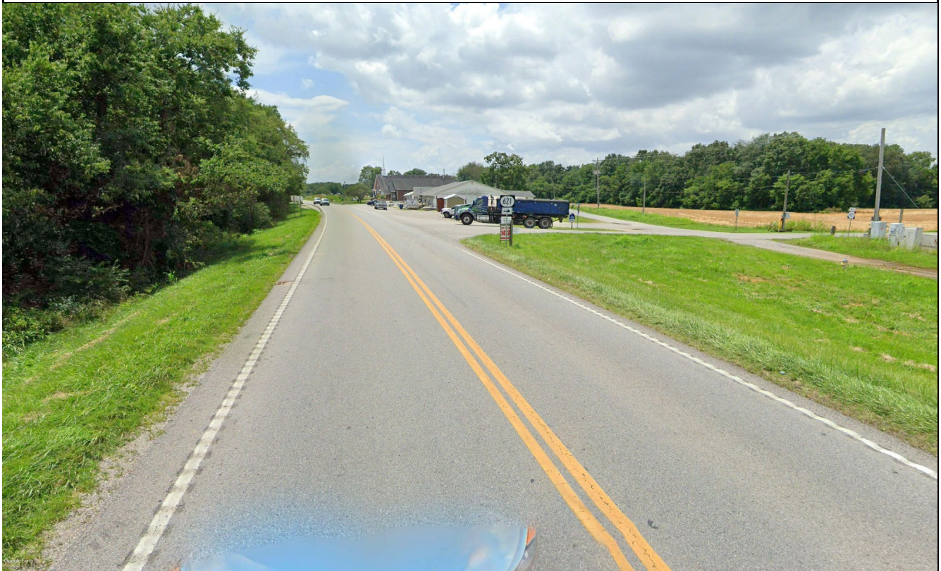
Two lane section of US 31W looking south near the intersection with KY 621
