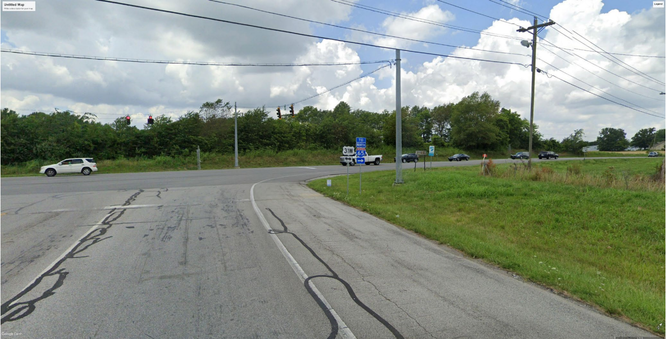
KY 1008 Intersection with US 31W. Project progresses to the right.
